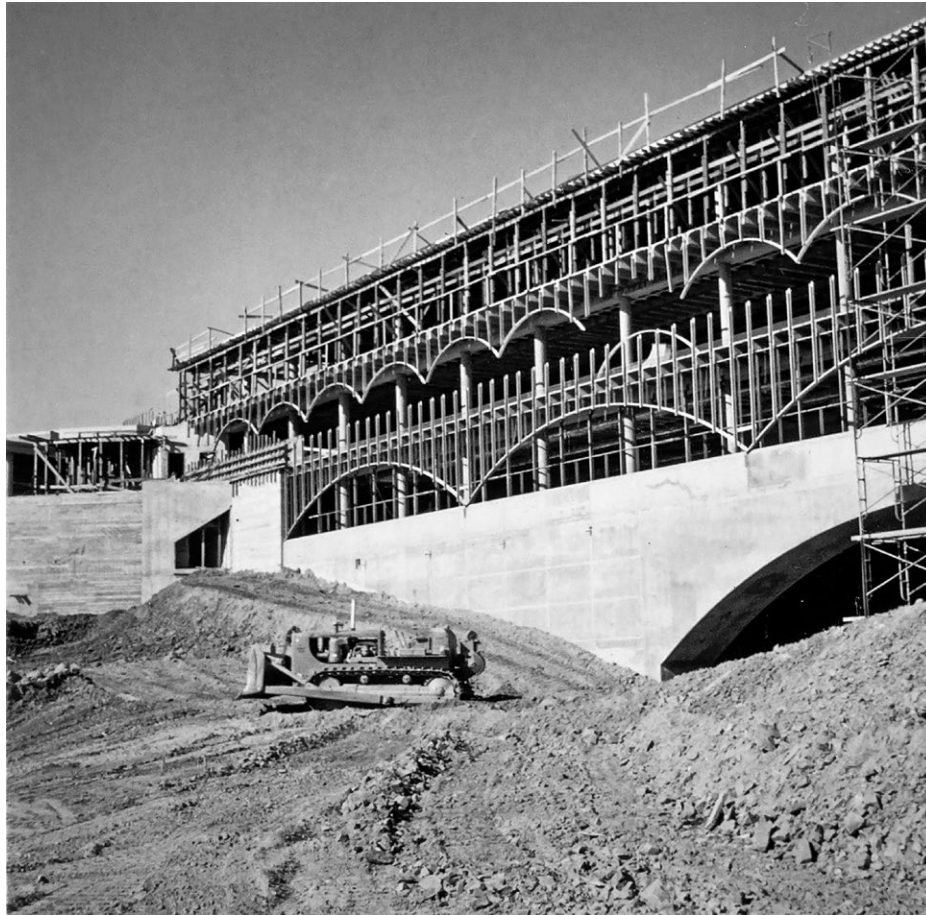
22 Frank Lloyd Wright, Marin County Civic Center, Administration Building, in construction, ca. 1960, viewed from the west with the library rotunda at left, showing the steel framework for plaster crescent arcs in front of columns on the second and third floors above the concrete arched base. The Frank Lloyd Wright Foundation Archives (The Museum of Modern Art | Avery Architectural & Fine Arts Library, Columbia University, New York), photograph no. 5746.0022 (photograph provided by The Frank Lloyd Wright Foundation Archives [The Museum of Modern Art | Avery Architectural & Fine Arts Library, Columbia University, New York])
