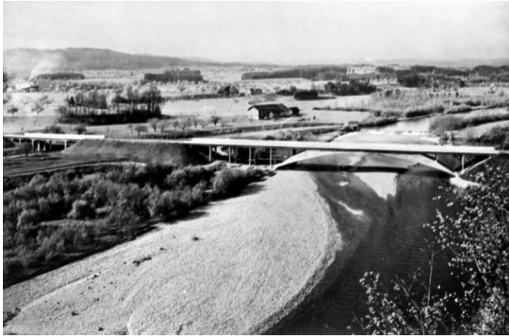
3 Robert Maillart, engineer, Bridge over Thur River near Felsegg, Canton Saint Gall, Switzerland, 1932–33, with the main span designed as a three-hinged arch. ETH-Bibliothek Zürich, Image Archive/Hs_1085-1933-3-13 /CCBY-SA 4.0 (photograph provided by ETH-Bibliothek Zürich)
